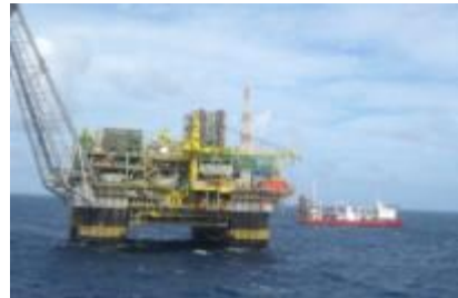
Roncador Field Development & P-52 Platform 1,800m water depth
