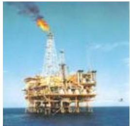
Garoupa Platform 1 st flexible pipe installed 100m water depth
