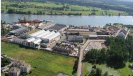
Flexi France: Le Trait, France World's largest Flexible pipe plant
