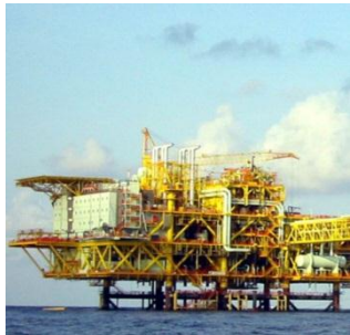
Conventional Fixed Platforms
