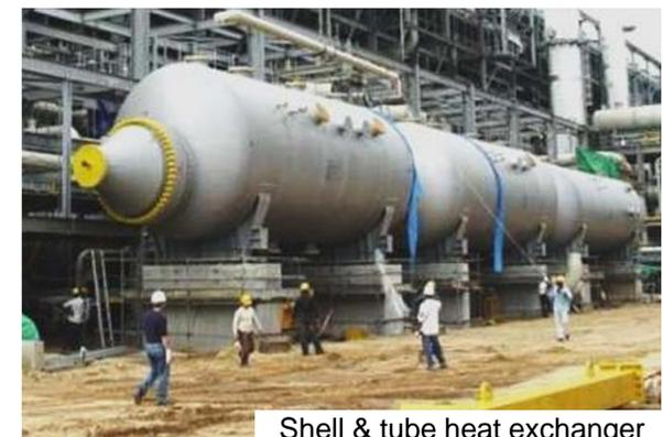
Shell & tube heat exchanger
