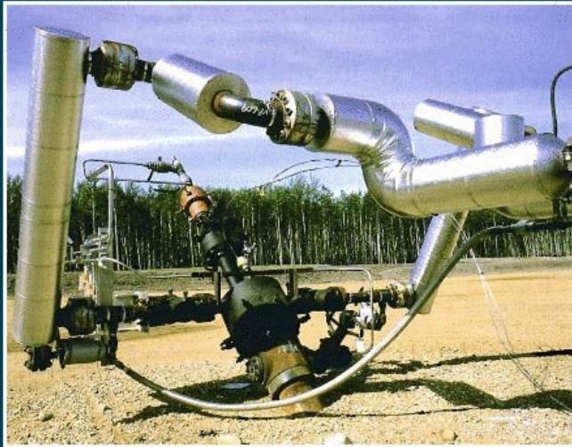
Oil Sands Thermal Wellhead
