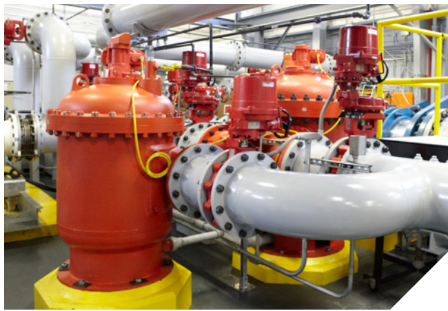
TechnipFMC Flow Research and Test Center
