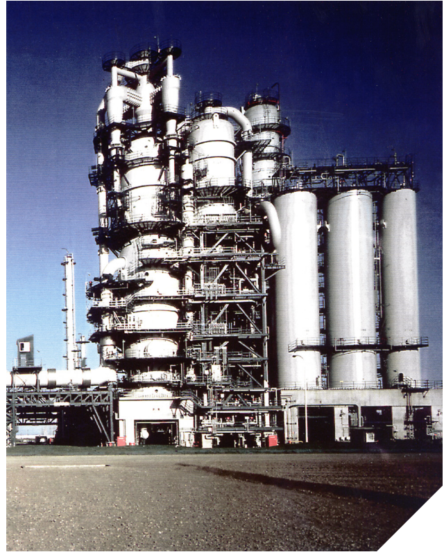
Hokkaido, Japan. This R2R Resid Cracker is designed for residue feeds up to 7.3wt% Concarbon at 32,000 BPD. (Photo courtesy Axens & Idemitsu)
